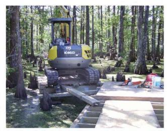
Previously installed walkway sections are used to support installing equipment without disturbing the environment.
