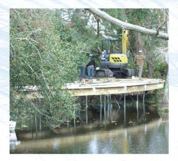
The flexibility of the helical piles permits the boardwalks to be built to best fit the environment, such as passing around tress.
